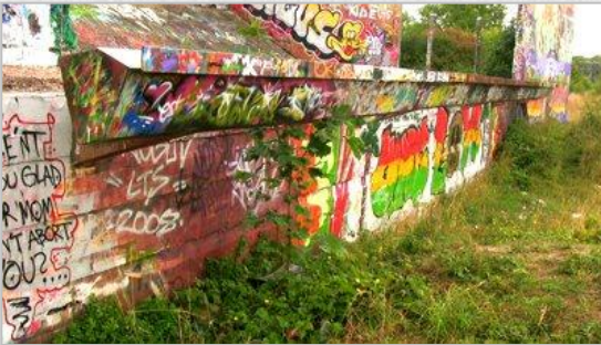
Retaining wall reinforced with concrete
