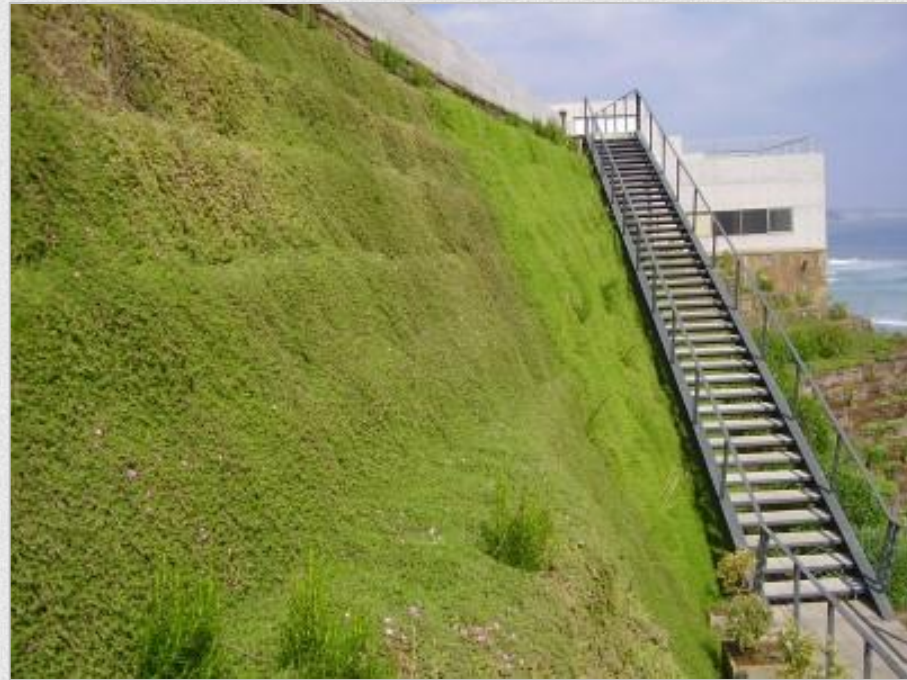
Soil wall reinforced with geosynthetics
