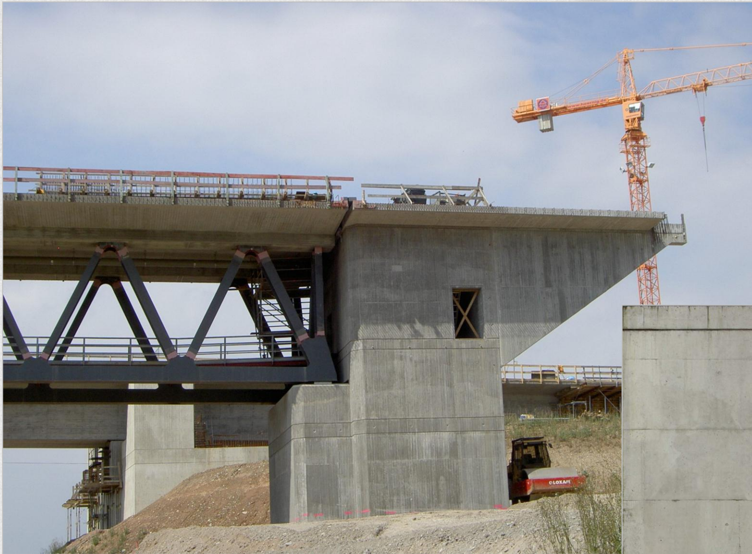
Bridge abutment reinforced concrete
