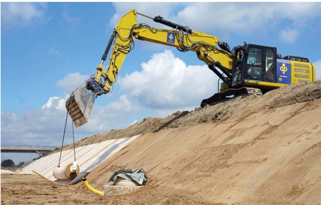
Figure 7 – Use of a bentonite mat to protect groundwater on the A33 motorway, Halle, Germany.
