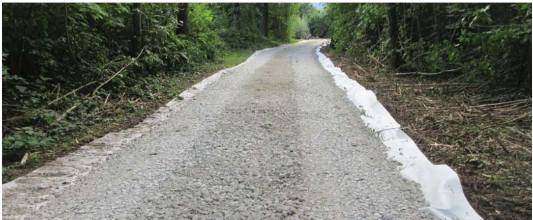
Figure 10 – Biodegradable nonwoven made from renewable raw materials as a separation and filter layer in a temporary construction road, Dettingen, Germany.
