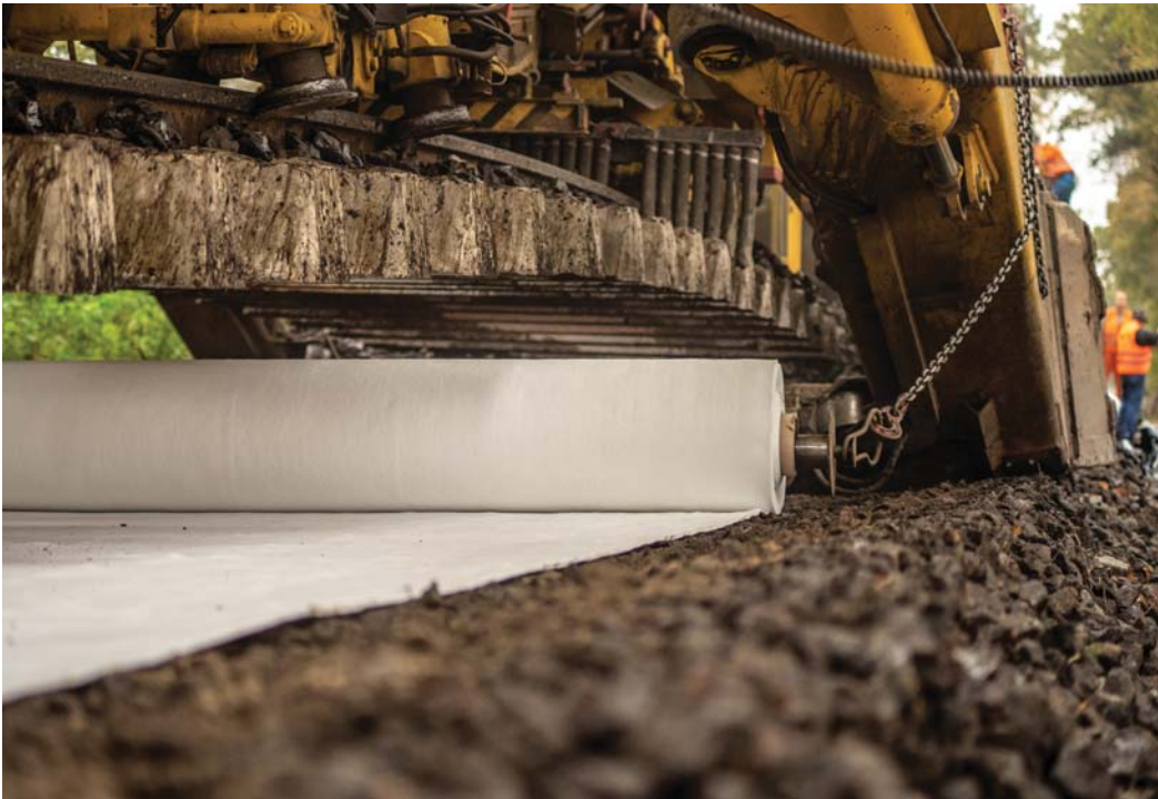
Figure 4 – Separating geotextile between the fine-grained subgrade and the coarse-grained base course layer in railway construction.
