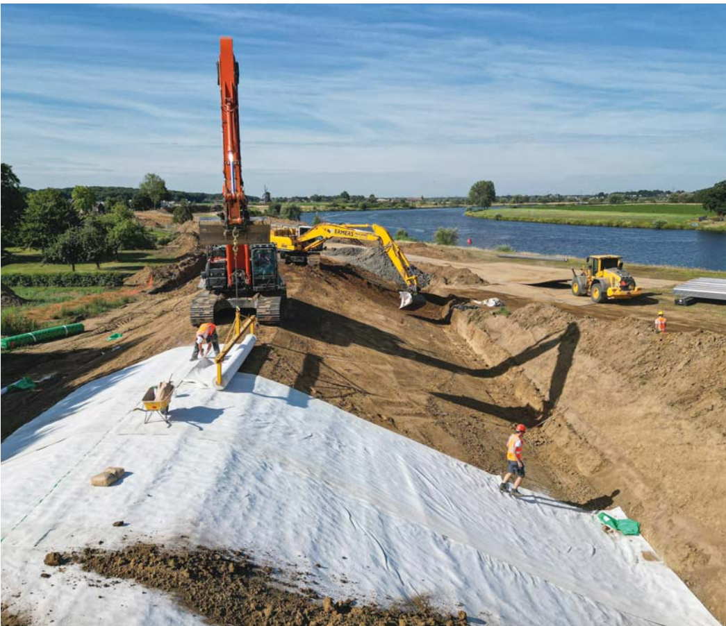
Figure 3 – Dyke improvement with installation of a bentonite mat on the crests and slopes of the flood defence to replace a full clay cover of 1 meter and stimulating re-use of local soil, Beesel, The Netherlands.
