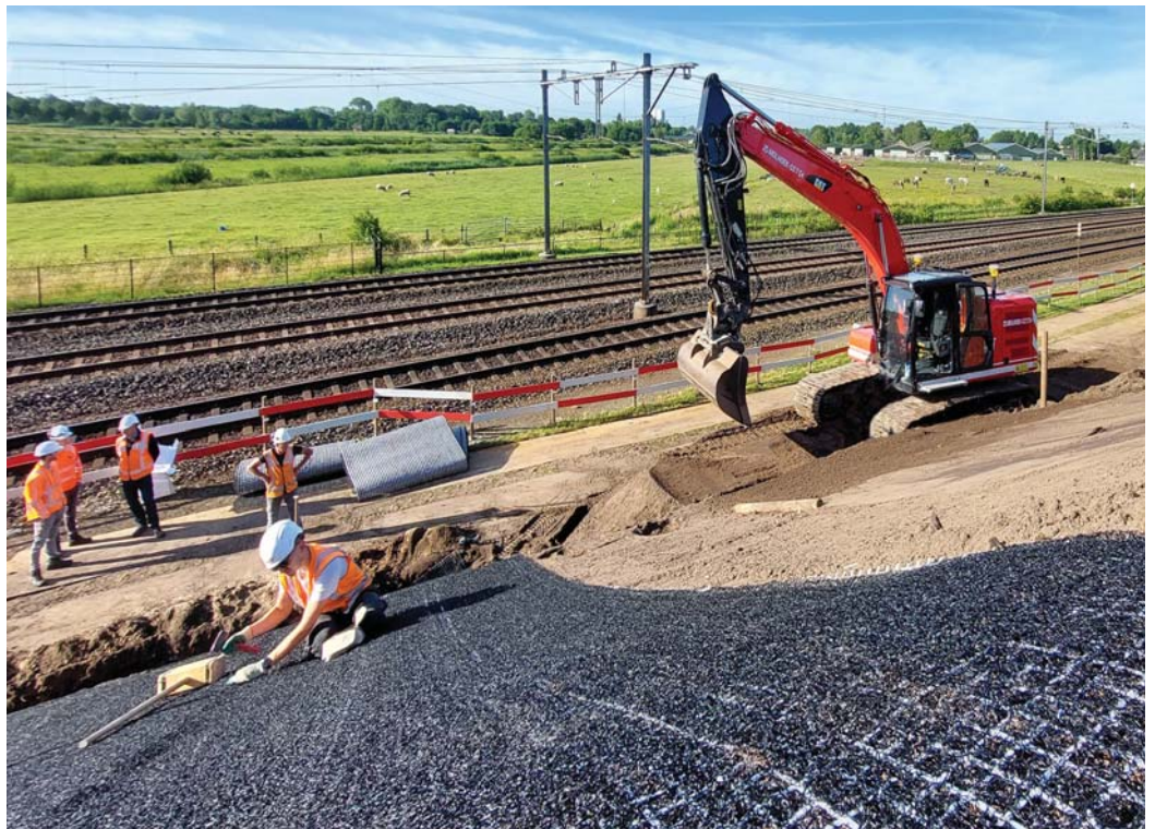
Figure 9 – Installation of a permanently reinforced erosion control system, securing an embankment slope next to a railway, Groenekan, The Netherlands.
