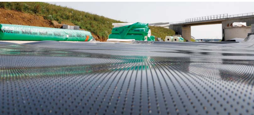
Figure 8 – Sealing the subsoil for groundwater protection with a HDPE geomembrane and nonwoven protection layers at the railway Wendlingen-Ulm parallel to the A8 federal highway, Germany.
