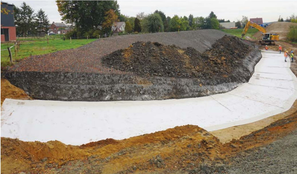
Figure 2 – Dyke foreland improvement with a bentonite mat creating sufficient length against the piping phenomena and meeting the Limburg Water Board design requirements for flood defence, Neer, The Netherlands.
